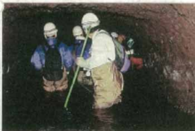
Inspecting the interior of the tunnel
