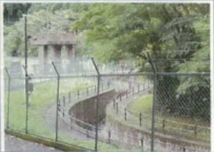
Sluice gate and Intake canal
