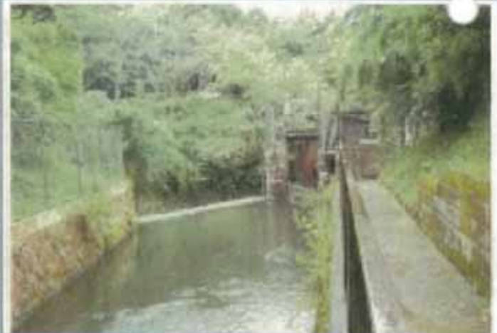
Looking downstream from the tunnel exit
