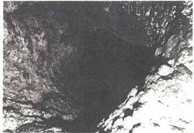
Shaft for Ventilation
