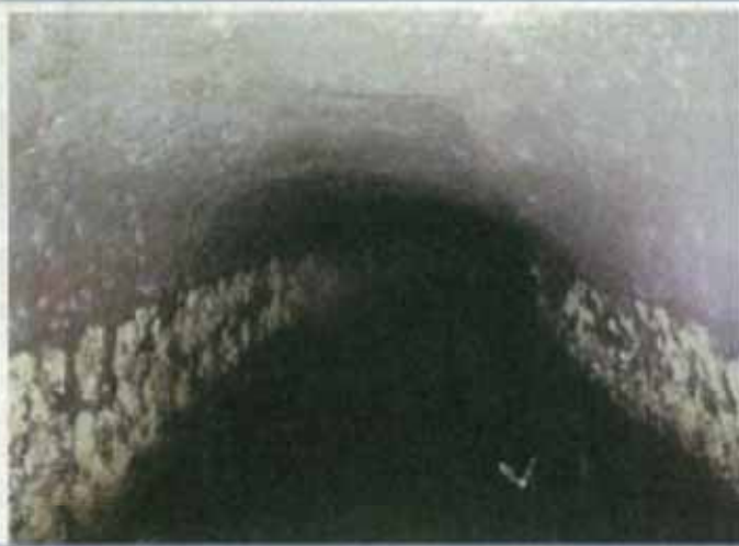
A horseshoe-shaped section of the tunnel where water flows gently
