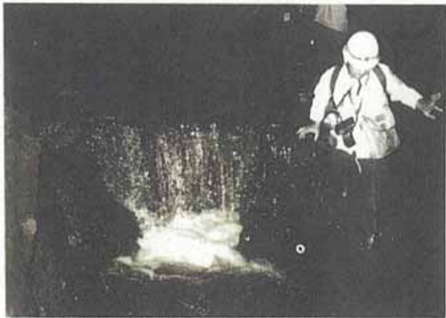
Drop at the Meeting Point of Tunnel Digging
