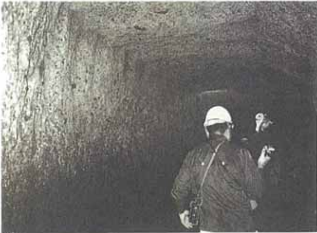
Interior of the Tunnel
